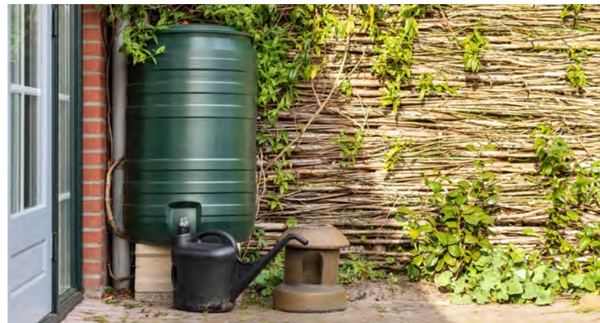
Water butt used to collect and store rainwater. Providing a sustainable source for watering plants during dry periods and reduces reliance on mains water.
